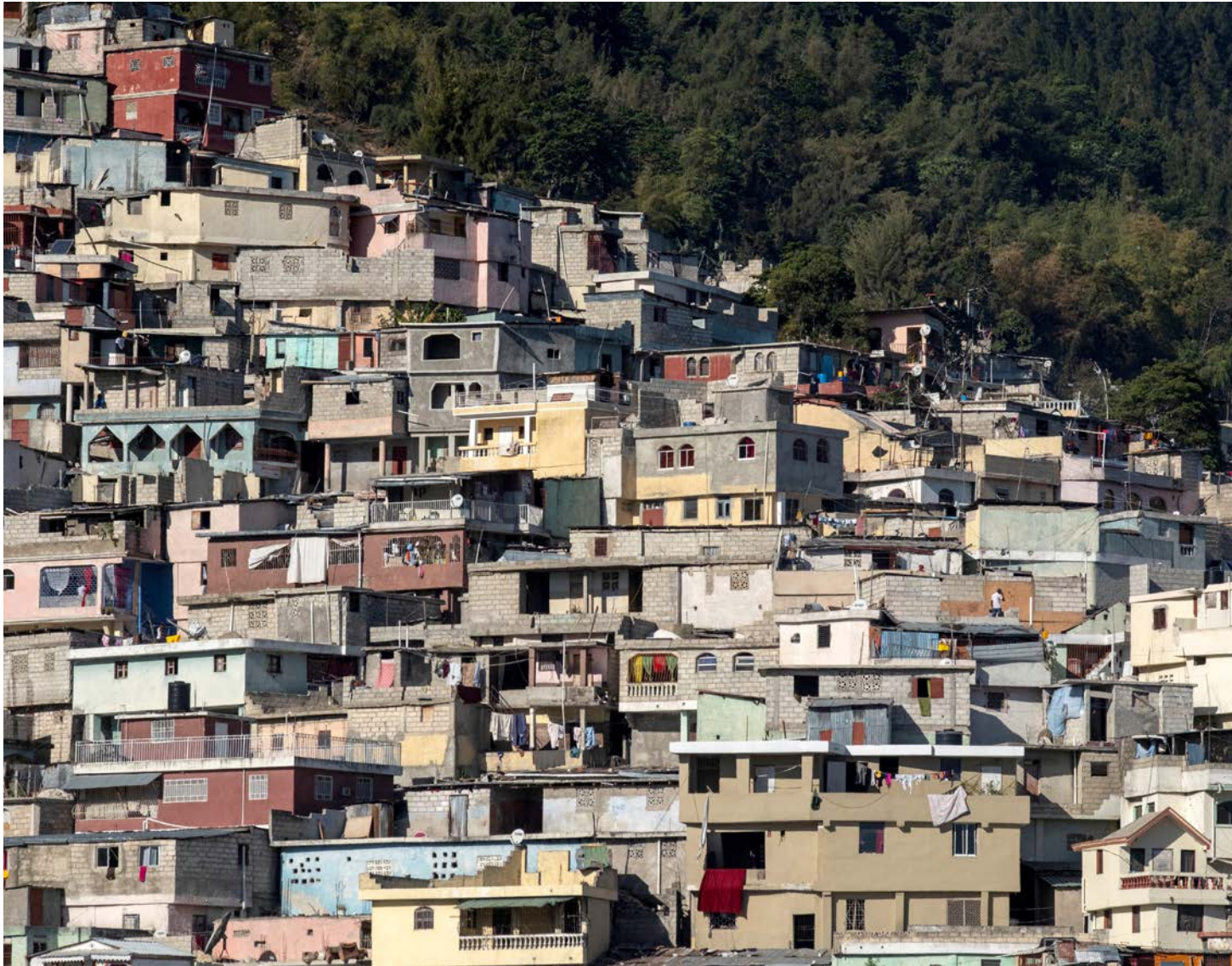
Steep decline: Jalousie district of Port-au-Prince, Haiti.
