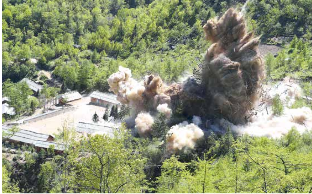
The process of implementing a thousand provisions starts with one blast: Detonation of the command post facilities of North Korea's nuclear test site in Punggye-ri.
